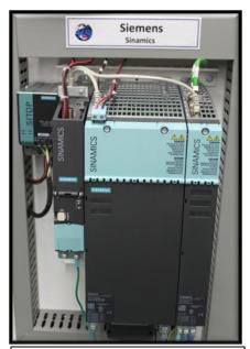
Sinamics System Consists of: • CU320-2 Control Module • 6SC3130 Smart Line Module • 6SL3120 Double Motor
