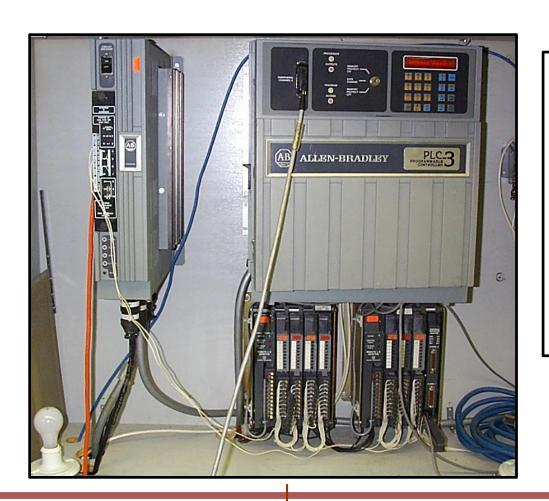
The PLC-3 and PLC-3/10 (1775 series) are a family of large programmable logic controllers. It is used primarily in the automobile industry where high reliability is essential to a good product. K+S guarantees this reliability by fully load testing all modules to their maximum capacity. This would include all memory modules and power supplies. Communication modules are tested in a closed loop system to ensure error free communication.
